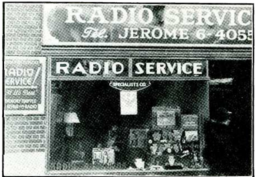
Foot-high letters blazon forth this shop's phone number. The neighborhood remembers, calls up when its sets go "haywire"
